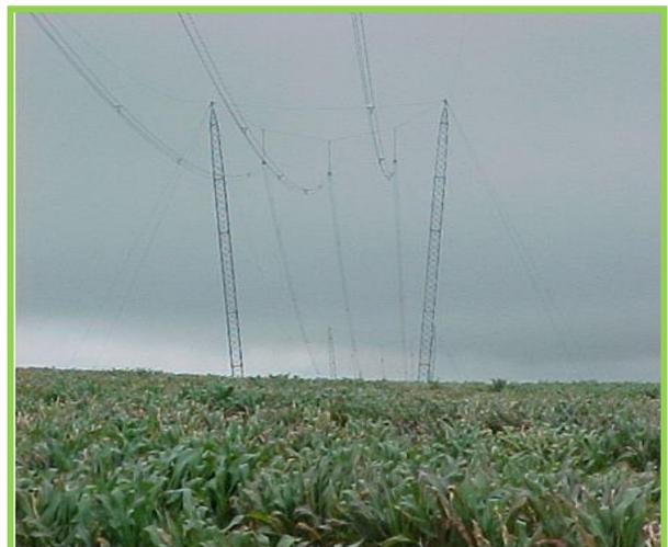
**Figure 9: Cross rope suspension tower.**
