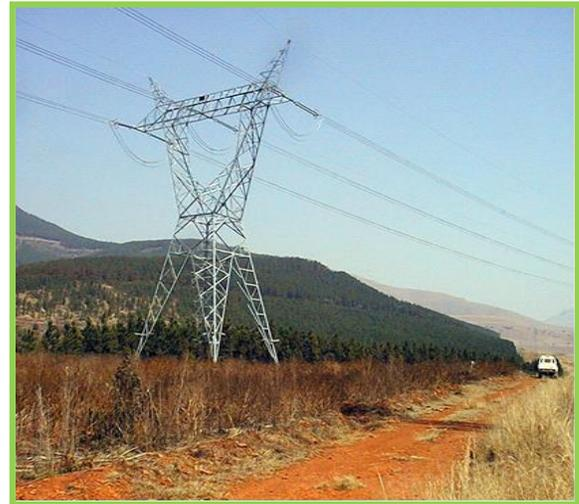
**Figure 12: Photographic illustration of Self-supporting suspension tower.**
